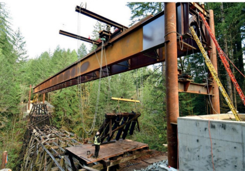
Once in place across Holt Creek, the new bridge became a working platform to disassemble the former timber crossing
