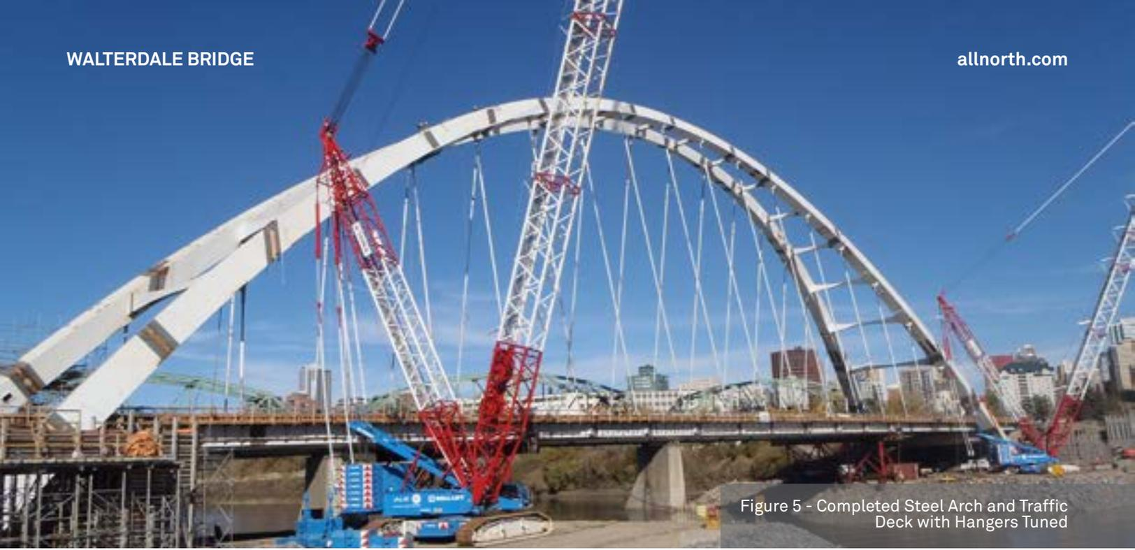
Figure 5 - Completed Steel Arch and Traffic Deck with Hangers Tuned
