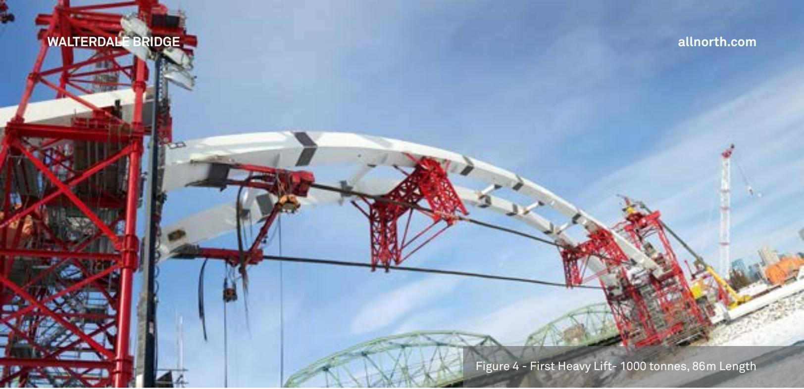
Figure 4 - First Heavy Lift- 1000 tonnes, 86m Length
